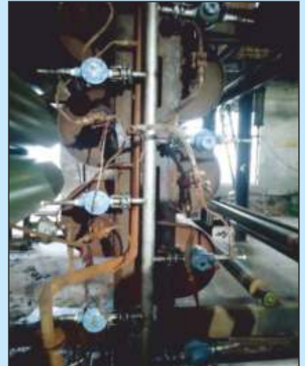
INSTALLATION OF BALL FLOAT TRAPS ON VERTICAL DRYING RANGE MACHINE (VDR) IN TEXTILE INDUSTRY
